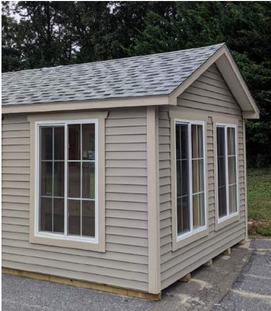
EXTERIOR FEATURING MIRATEC TRIM
